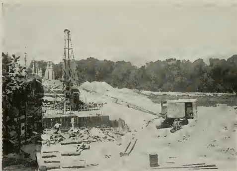
Northwest Caterpillar at Pier. Old Bridge at Left.
